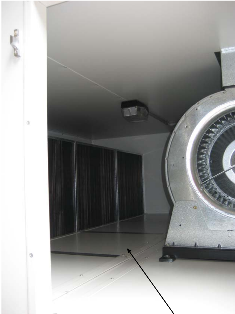
Removable Panels for Coil Access
