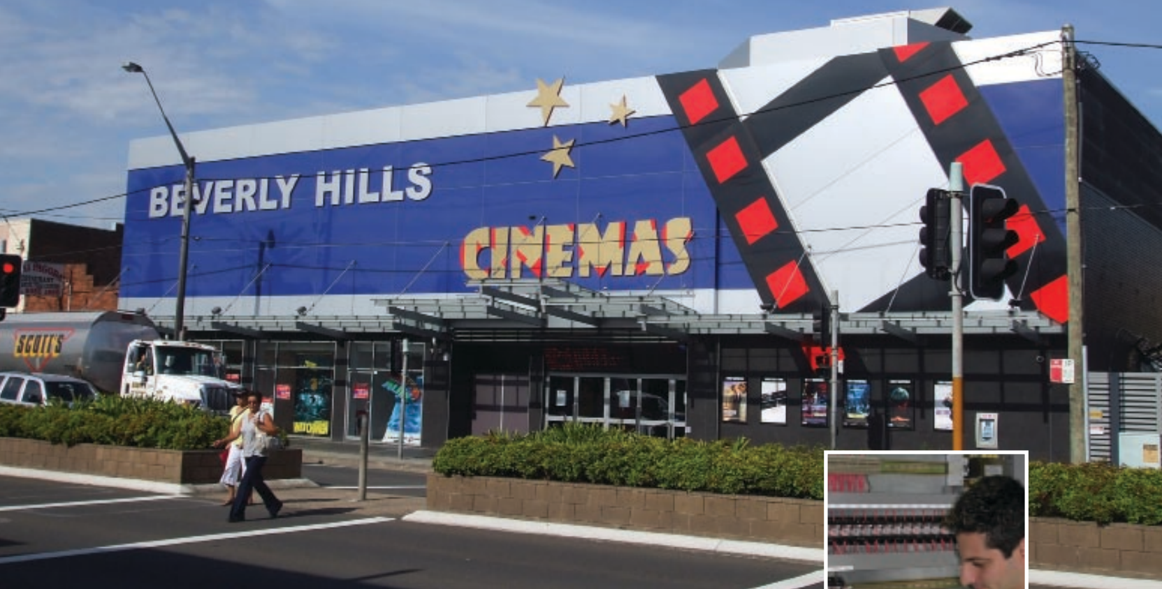
Beverly Hills Cinema complex with AC system visible on the roof. Inset: Engineer George Kyprianou checks the temperature control.
